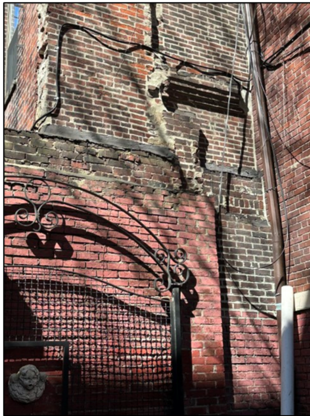
Figure 23. Detail of abutting brick walls at park-side elevation.
