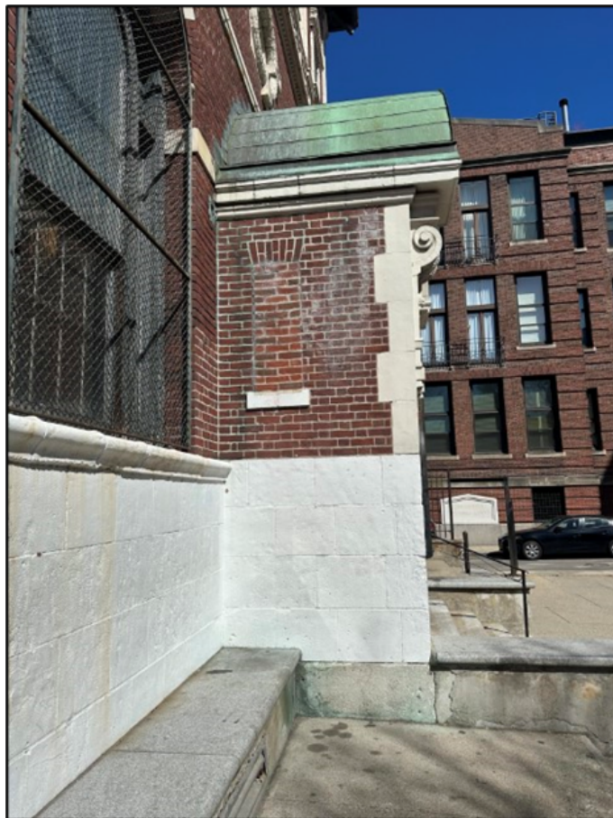
Figure 8. Side view of front entrance.
