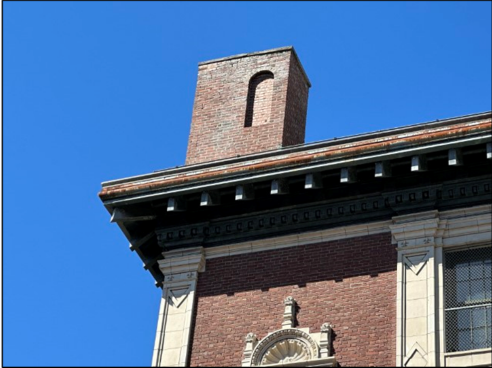
Figure 9. Façade view of cornice and chimney.
