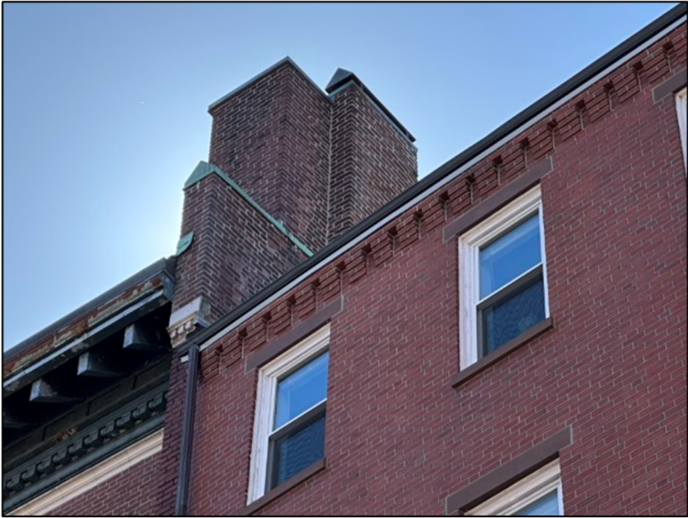
Figure 16. Chimney, cornice, and brick dentil elements.
