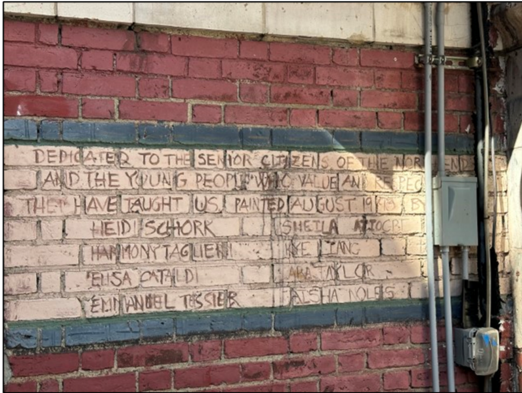
Figure 21. Brick detail on park-side elevation.
