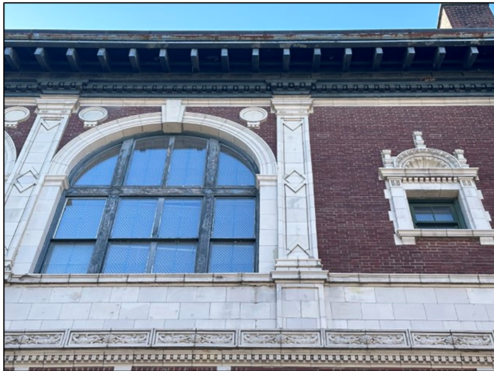
Figure 11. Rounded arched window at the North Bennet elevation.
