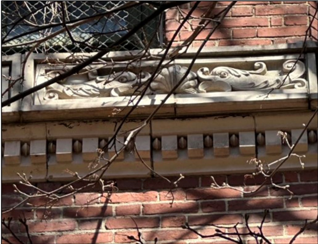
Figure 20. Detail of park-side elevation frieze.
