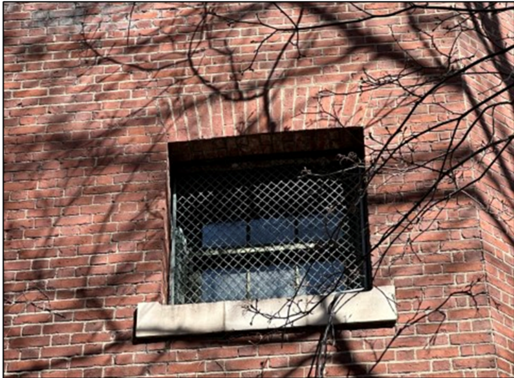
Figure 22. Small window on park-side elevation.
